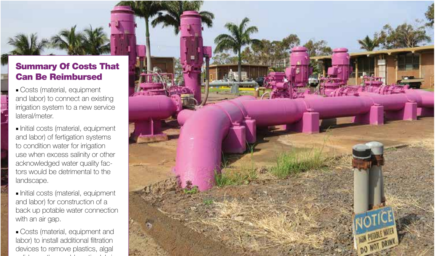
“Safety Purple” aka “OSHA Purple” is the required color for piping and fixtures for R1 water. The official color designation is Pantone 512.
